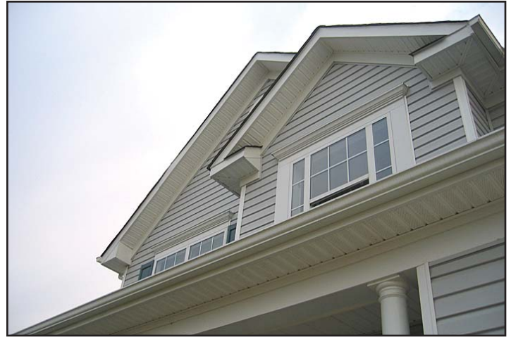
Electrical licensing and inspection rules do apply to siding replacement work when items such as luminaires, receptacle outlets and utility load-shedding devices must be removed and reinstalled.
